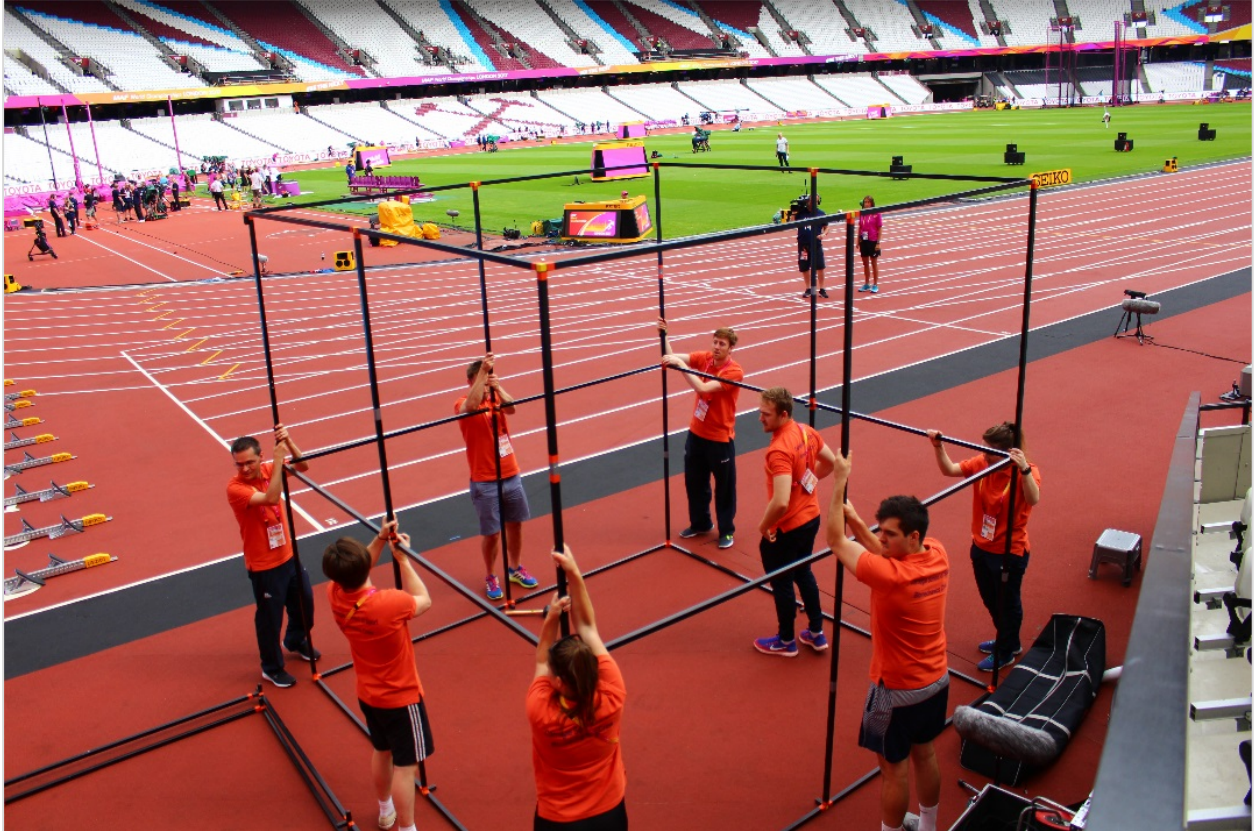
Figure 2. Discus calibration frame during construction at the London Stadium.
